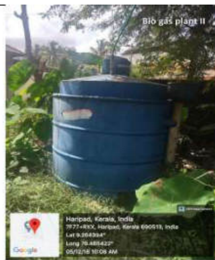
Biogas Plant II
