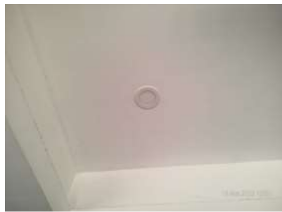
Image 3.e : Energy efficient LED lights in Waiting Area
